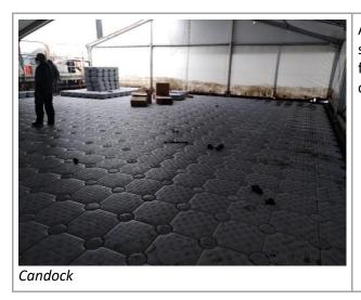
A floating pontoon is being installed. Aerosol spreading is significantly reduced. Limited aerosol formation can be observed along the edges of the cover.
